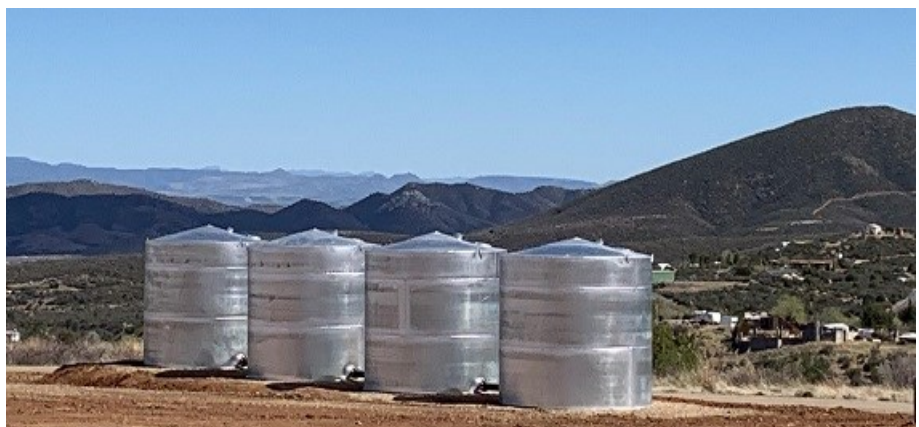
Four BIG water tanks are in place, thanks to the help of many, including the generous donation of CAFMA.
