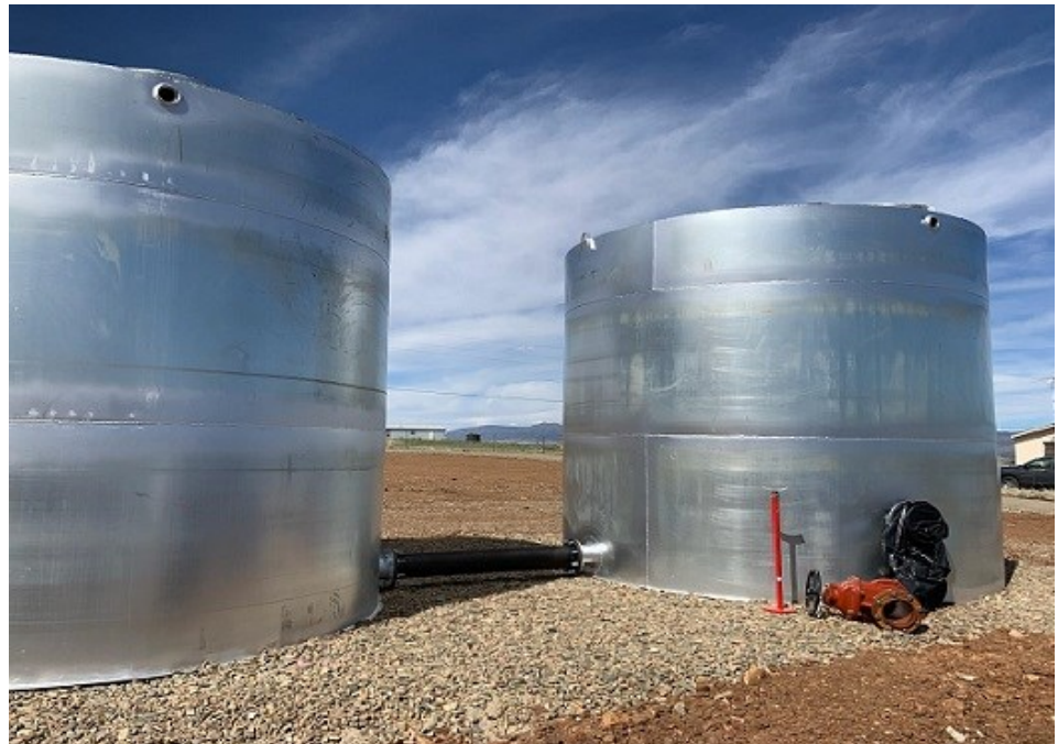
Installment underway! April 8, 2019.
