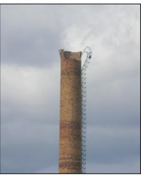
The recent monsoon has caused the remaining Humboldt Smelter stack and flue chamber to start failing. Another section of the top of stack has fallen. The only thing holding up the stack right now is the ladder and the last of the flue chamber. If the rest of the flue chamber falls, the stack will go with it.
