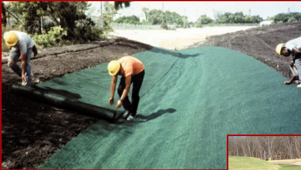
TURF REINFORCED MAT)
