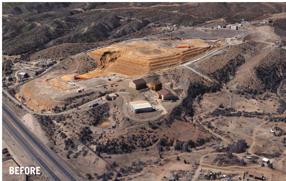
Figure 15A. Former Iron King Mine tailings pile before cleanup.
