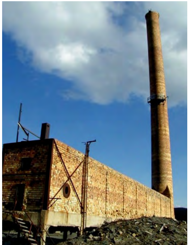
Former brick Humboldt Smelter stack and converter flue building on the smelter plateau.
