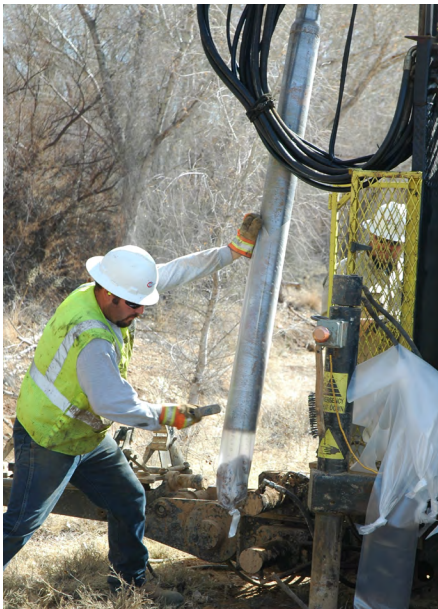
Field workers collect a core from a soil boring in the tailings flood plain.
