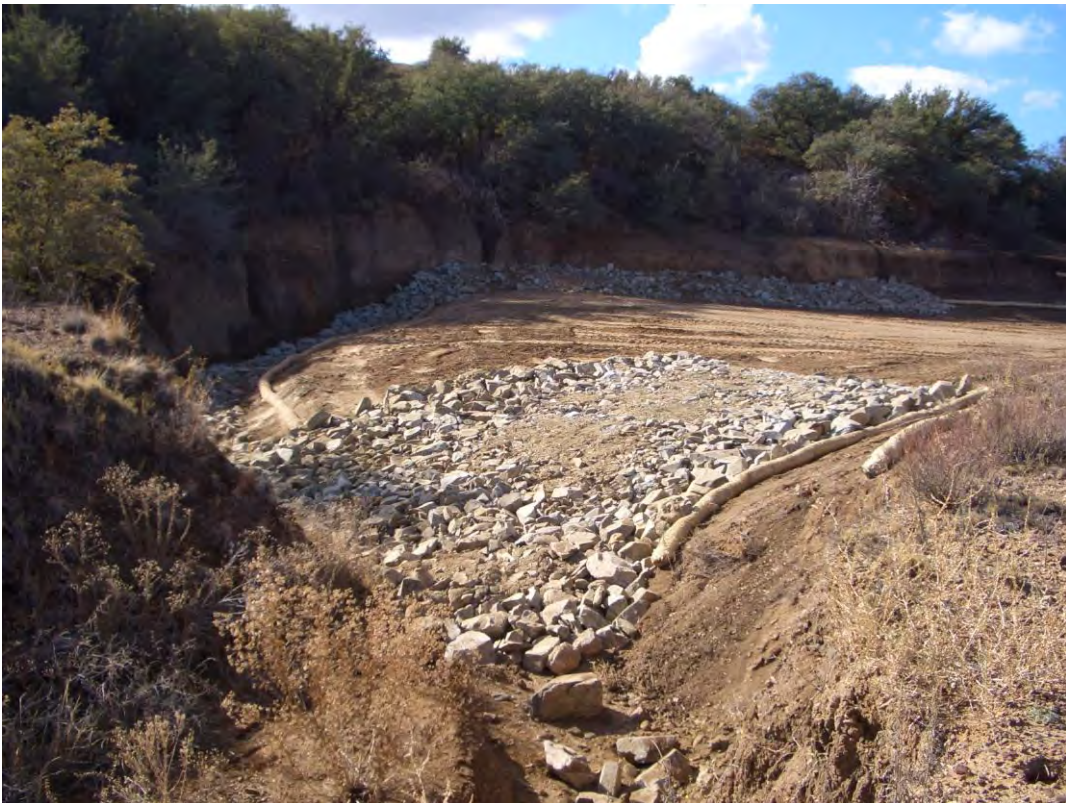
Final riprap-lined outfall leading into the south gully
