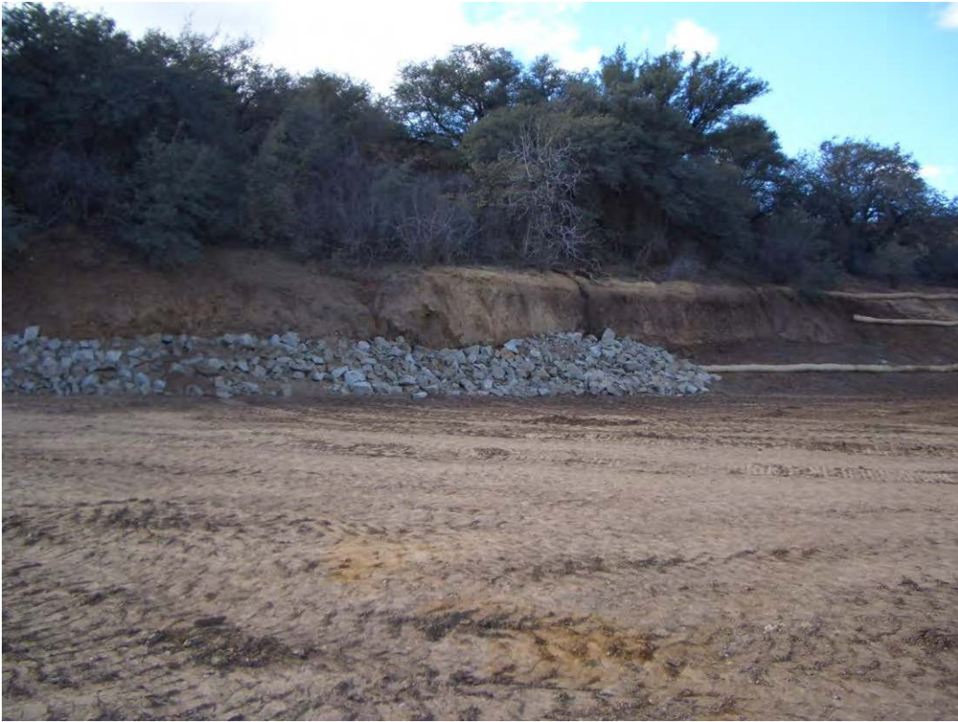
Vertical embankment with final riprap buttress
