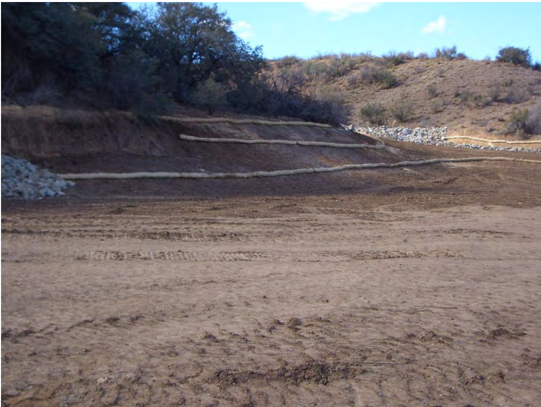
Final graded slopes with straw wattles
