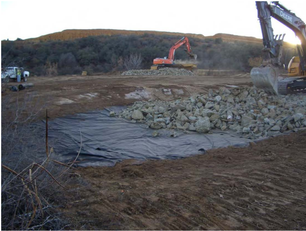
Construction of downstream stilling basin
