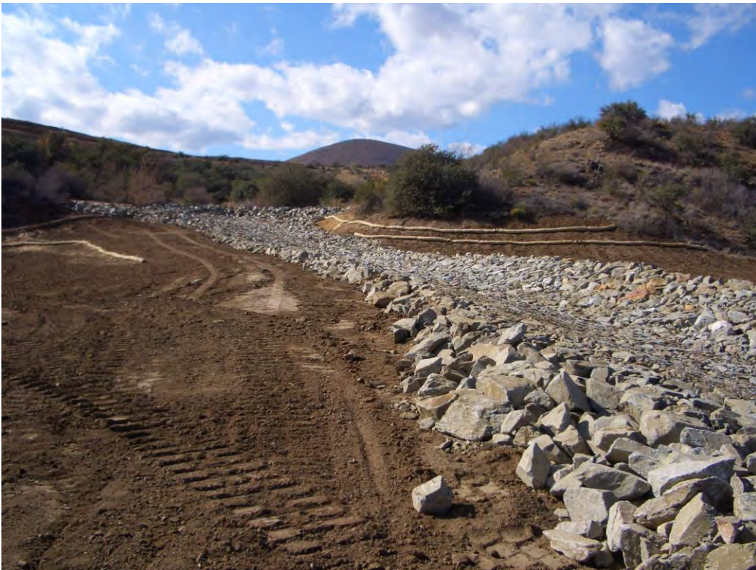
Completed channel section, looking upstream
