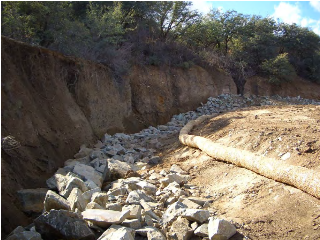
South gully – after grading and riprap treatment
