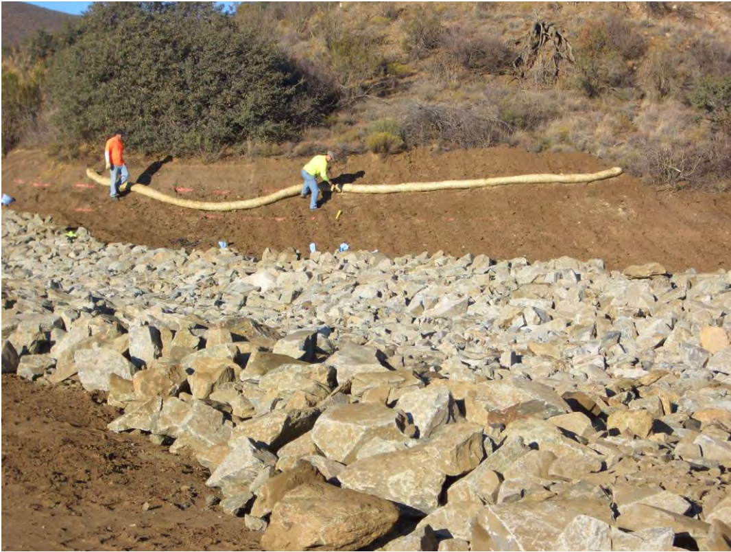
Installation of straw wattles along slopes
