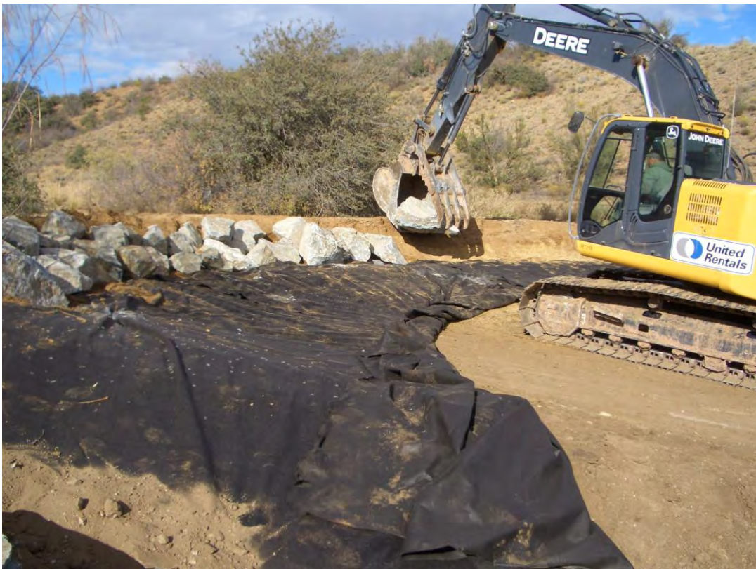
NP area – beginning of riprap treatment
