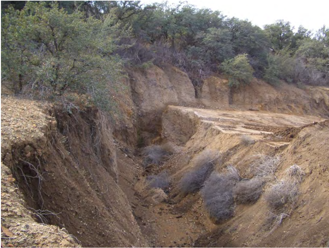
South gully prior to final grading
