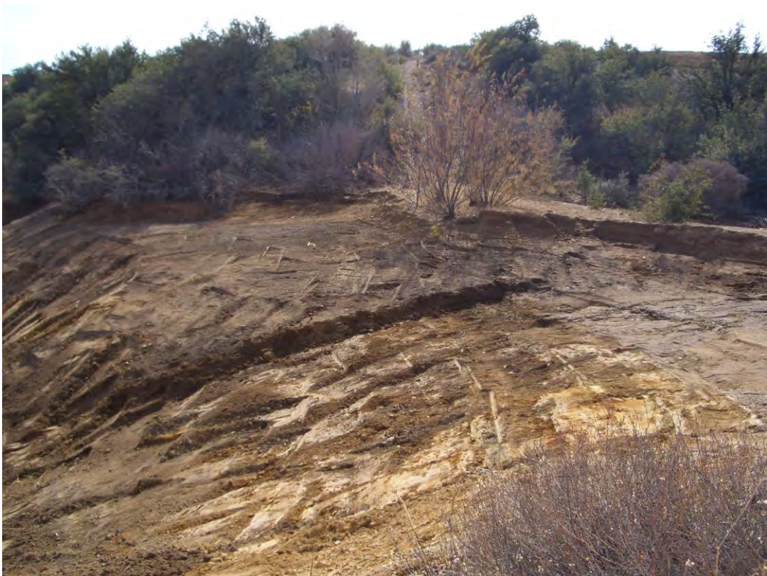
NP area prior to final slope adjustment and grading
