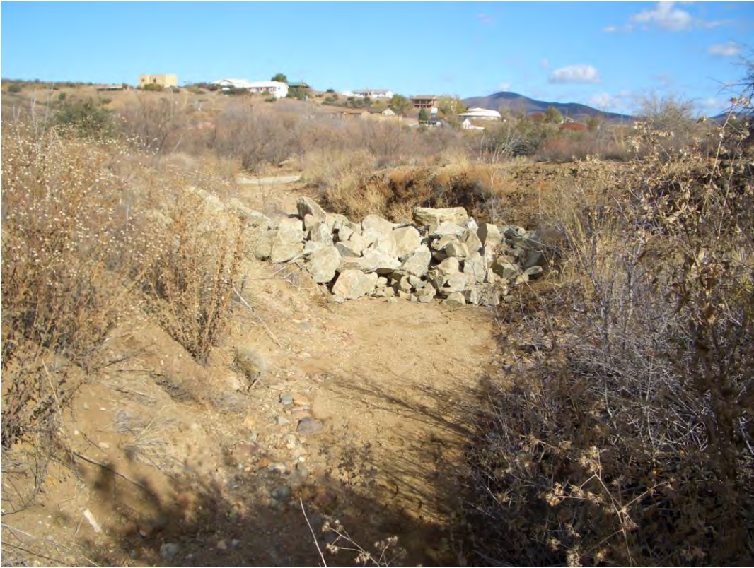
Rock check dam along downstream section of the south gully
