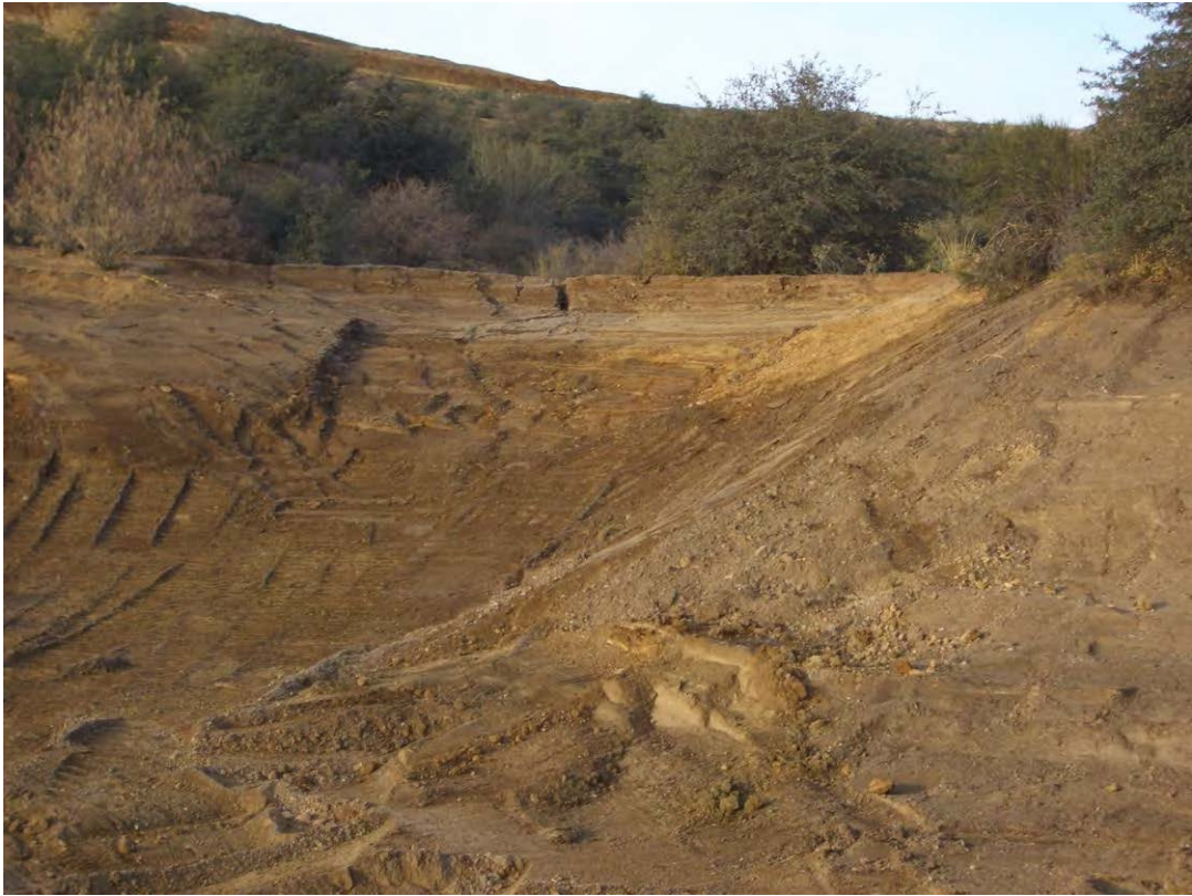
Nickpoint (NP) area prior to final slope adjustment and grading
