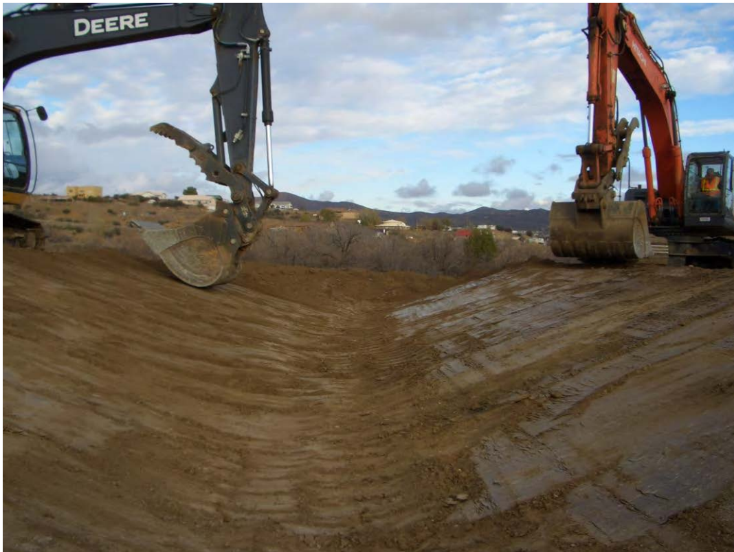
Diversion channel excavation and shaping
