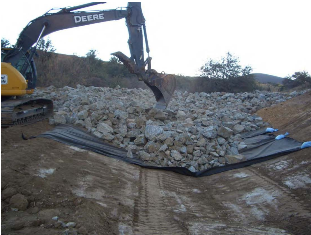
Completed NP area, looking upstream
