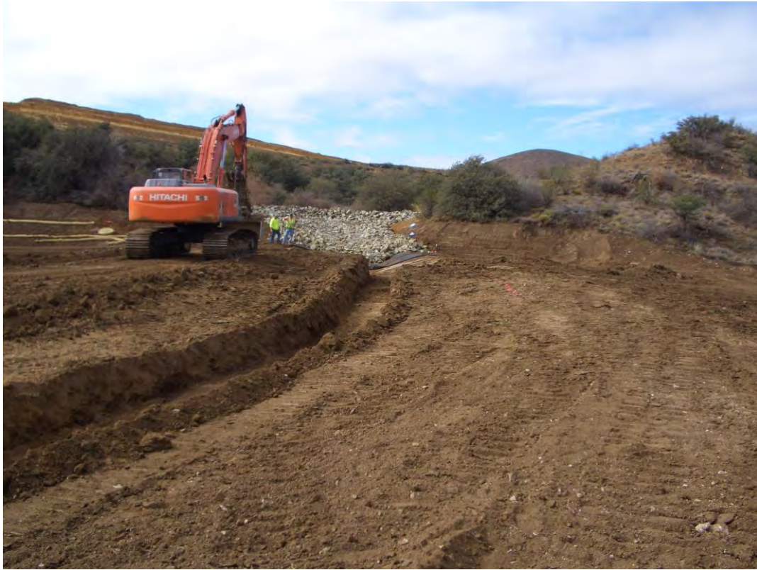
Excavated centerline of diversion channel, downstream of NP area
