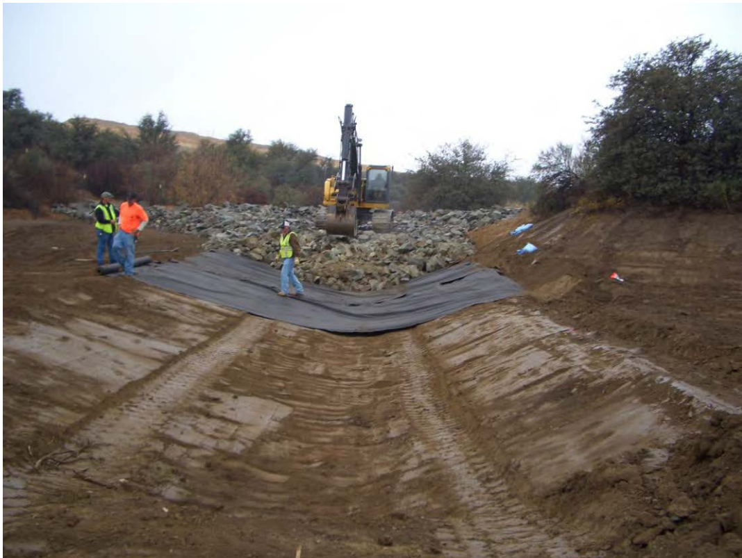
Diversion channel construction, downstream of NP area
