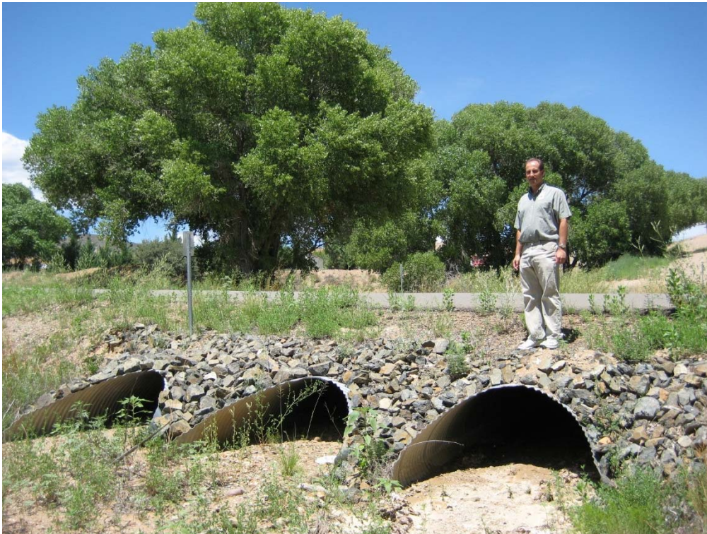
Photograph 10: Chaparral Gulch at 3rd Street, downstream of Highway 69 at VP9. Photograph taken in 2008; additional alluvium (from other sources in the drainage basin) has been deposited at this VP in recent years.
