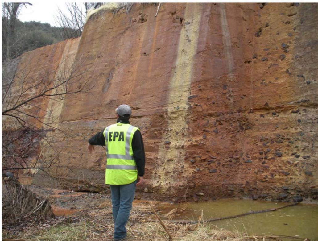
Photo F002 DSCN0939: Chaparral Gulch Dam
