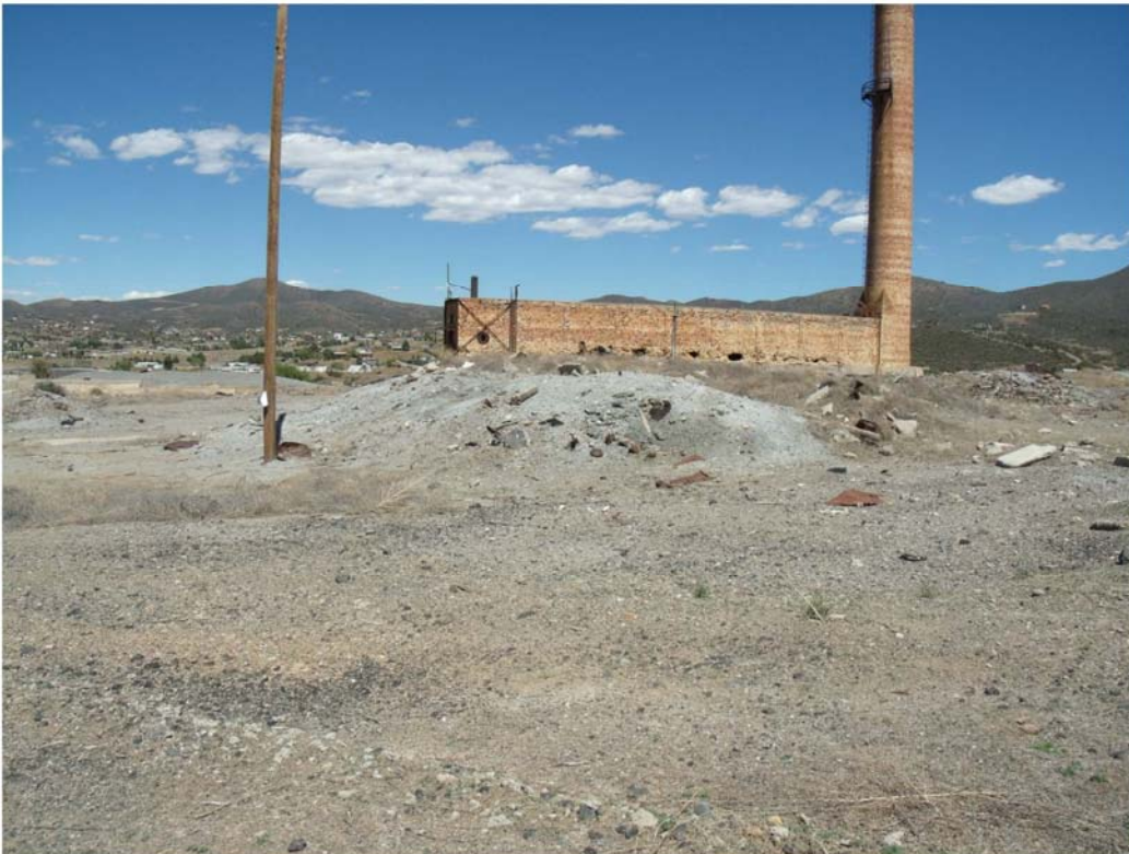
Photo GEDC1490: Dross material covering Pyrometallurgical Operations area at Humboldt Smelter
