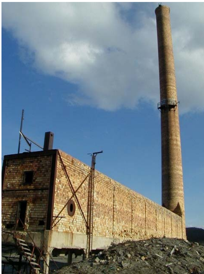
Photograph 26: Former Humboldt Smelter Pyrometallurgical Operations area, Smelter Stack and brick flue at VP24
