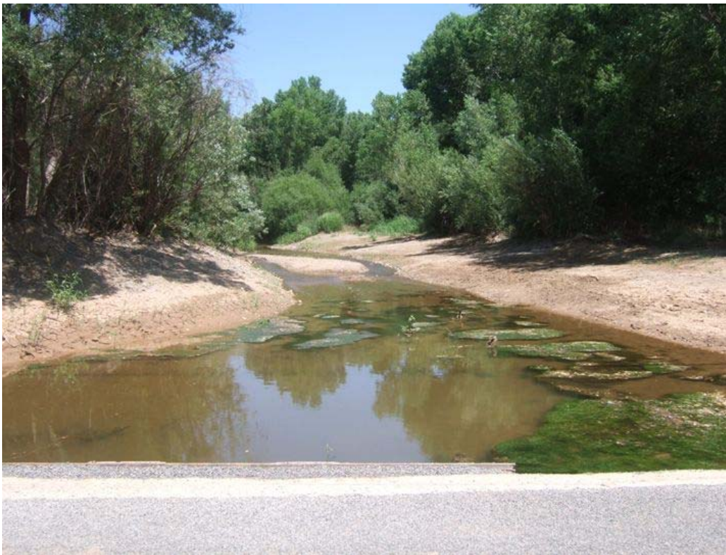
Photograph 36: Agua Fria River at Prescott Street, looking north at VP31
