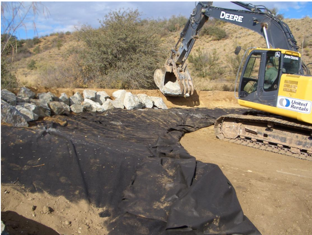
NP area – beginning of riprap treatment
