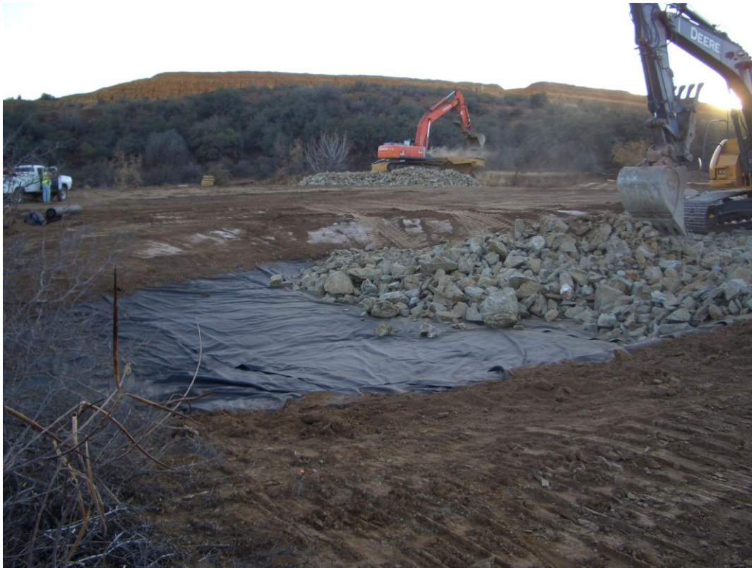
Construction of downstream stilling basin
