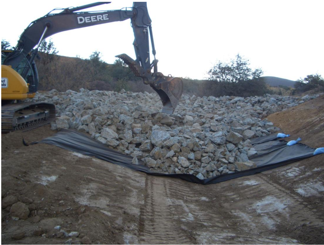
Completed NP area, looking upstream
