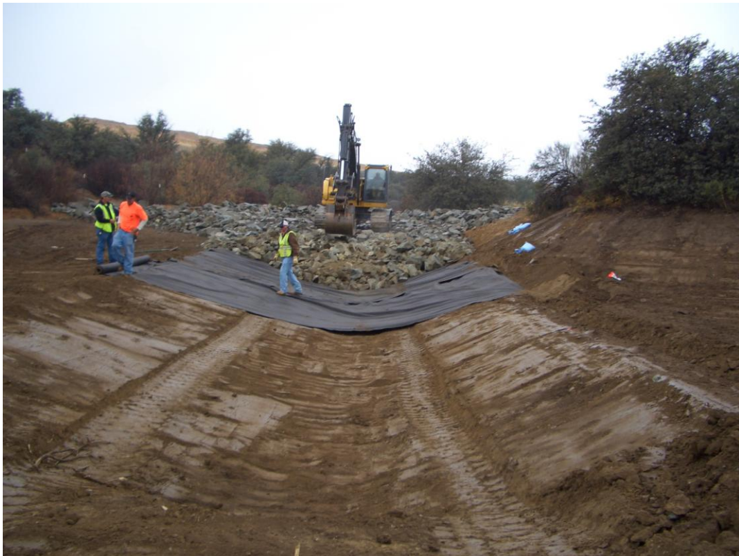
Diversion channel construction, downstream of NP area
