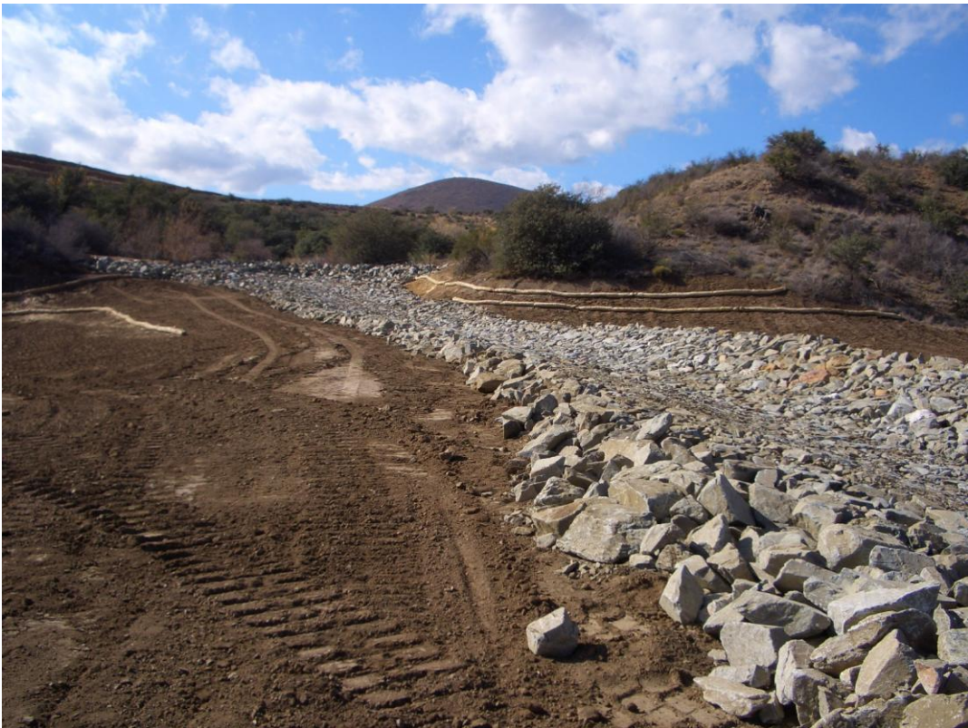
Completed channel section, looking upstream
