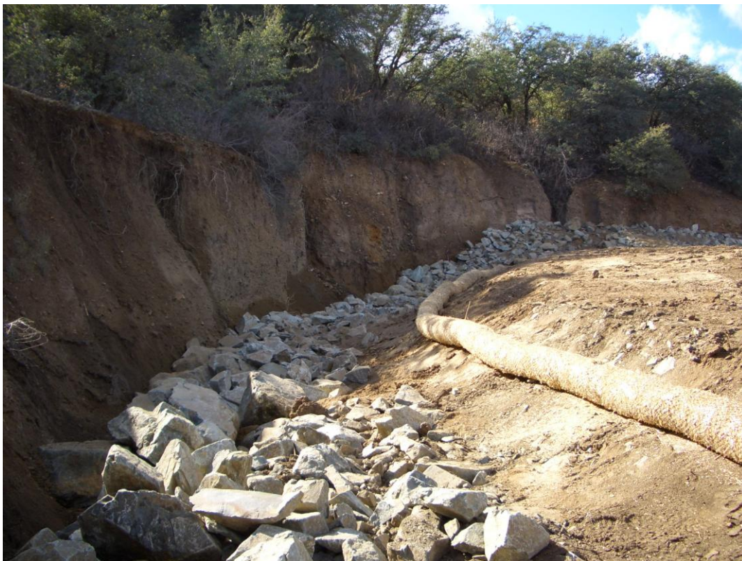
South gully – after grading and riprap treatment
