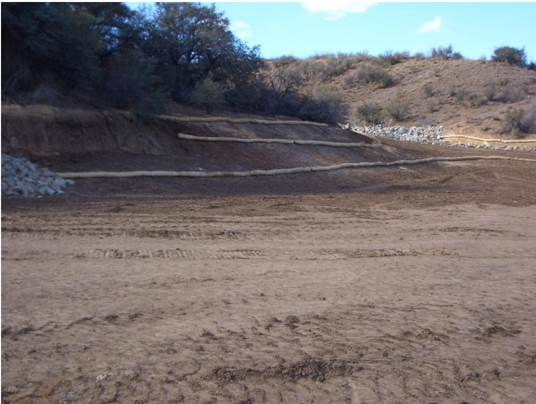
Final graded slopes with straw wattles
