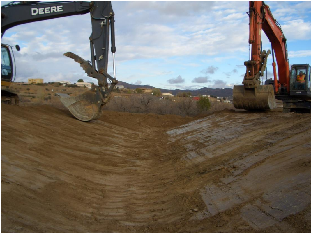
Diversion channel excavation and shaping
