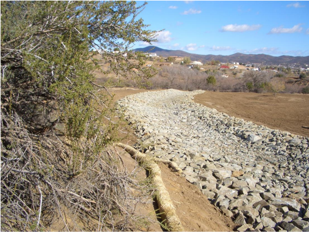
Completed diversion channel, looking downstream from NP area
