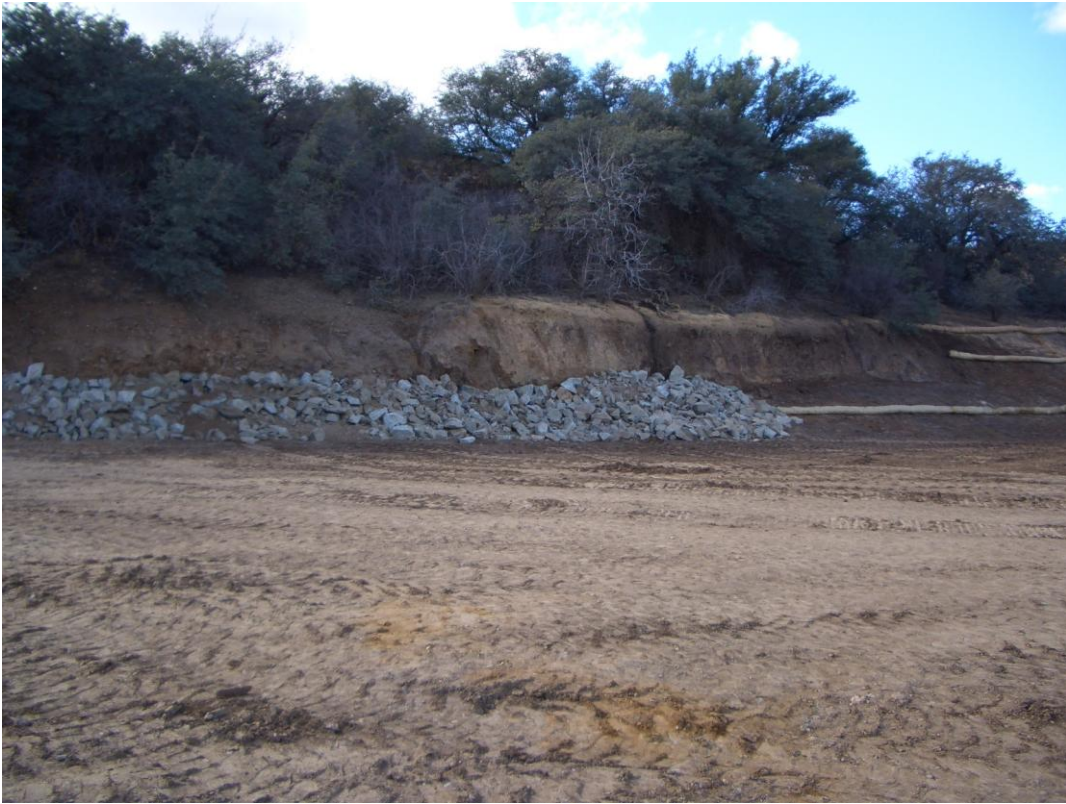
Vertical embankment with final riprap buttress
