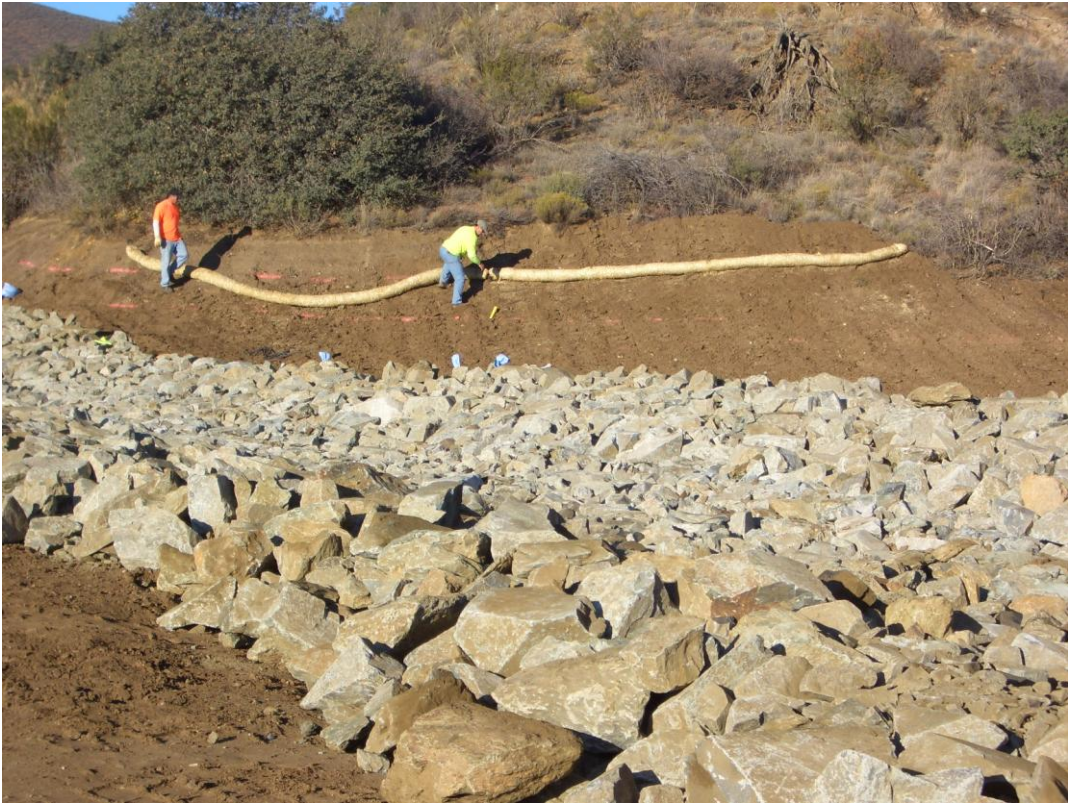
Installation of straw wattles along slopes
